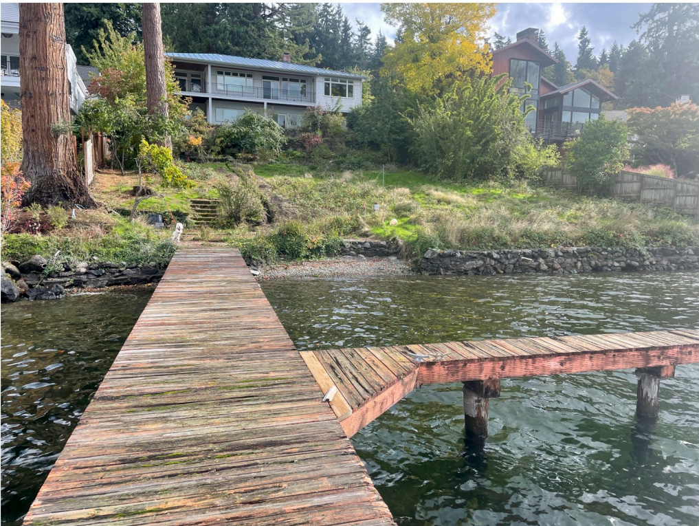
Photo 2 - Existing dock looking landward.
