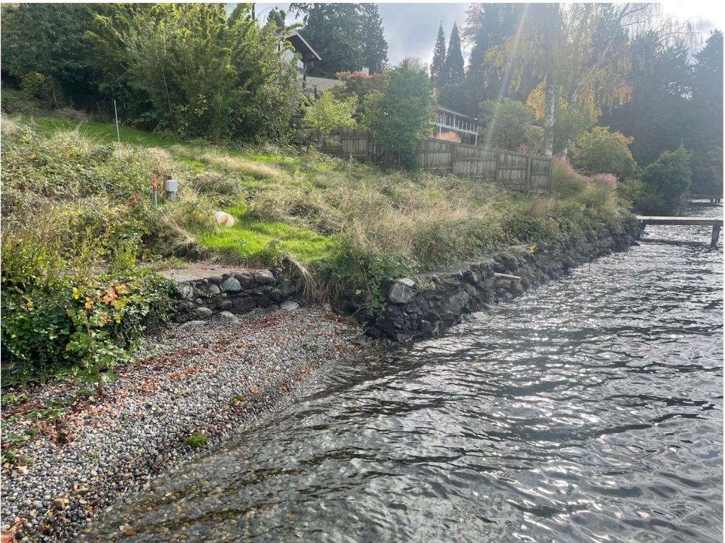
Photo 4 - Existing shoreline looking south.
